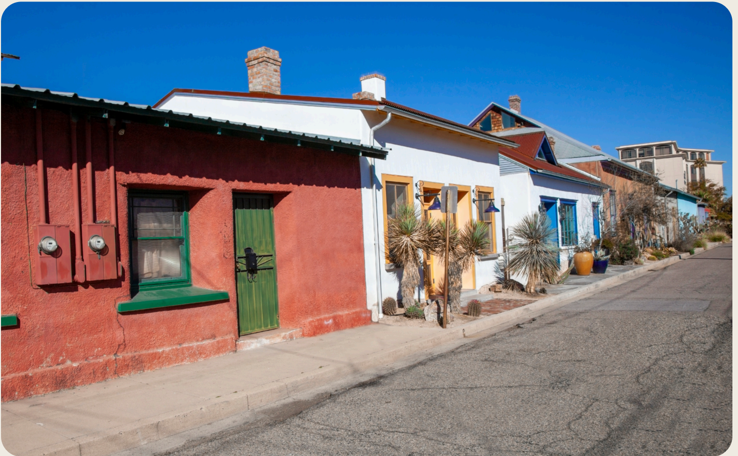
Colorful adobe homes line a sunlit street in Tucson’s historic Barrio Viejo district. Photo courtesy of Adobe Stock.
